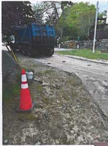
Replacing walk after installation of sewer line at O'Neill
