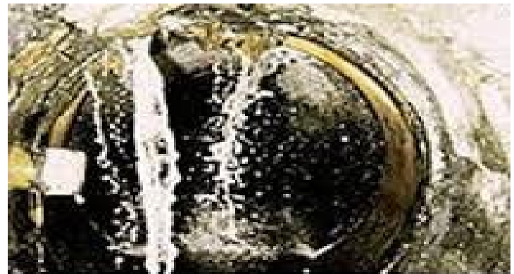
Examples of CCTV footage of Infiltration from faulty pipe joints
