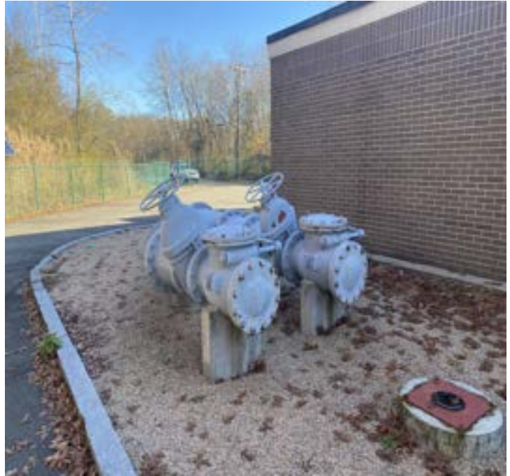
Emergency By-Pass Discharge Piping
