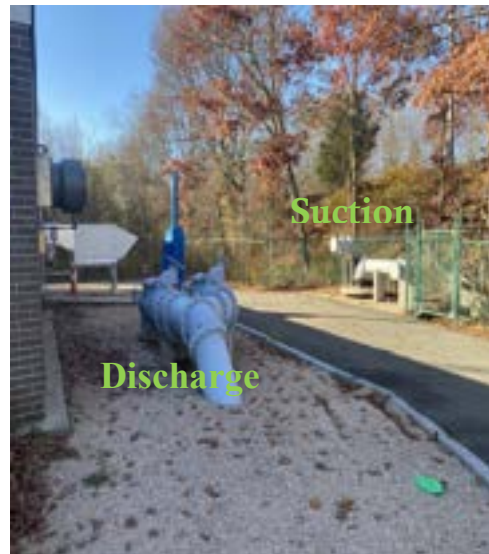
The pump would be temporarily installed between Suction and discharge piping in event of station failure.
