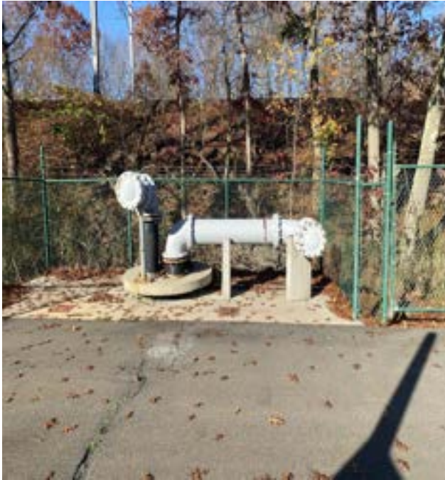
Emergency By-Pass Suction Piping
