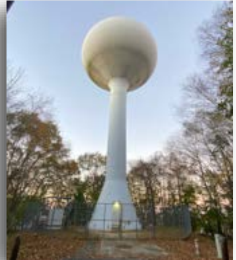
Vauxhall Street Water Tower Built 1973 - Rehab 2003 Capacity – 300,000 Gallons
