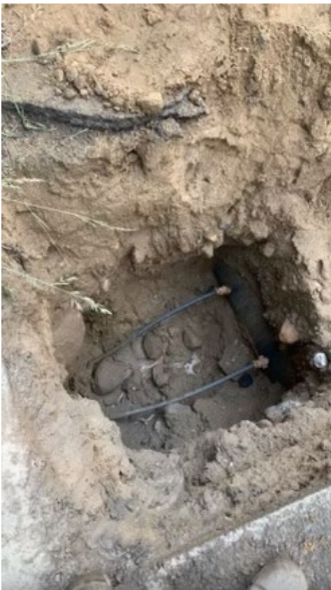
Plastic Water Service prior to replacement
