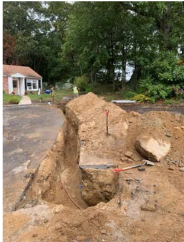
Plastic Water Service replaced with copper line
