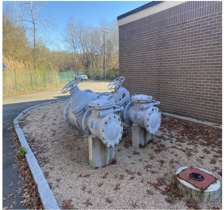
Emergency By-Pass Discharge Piping
