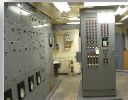
Pump station motor control panel.
