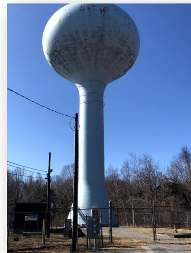
Fargo Lane Water Tower Built 1986 Capacity– 750,000 Gallons
