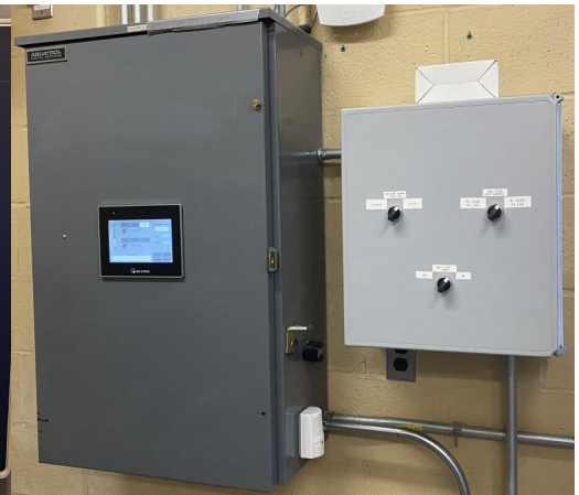
Redundant Level Control System
