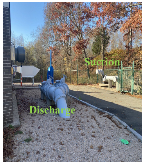
Pump would be temporarily installed between Suction and discharge piping in event of station failure.
