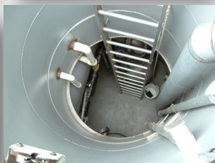
Access to bottom of pump station.
