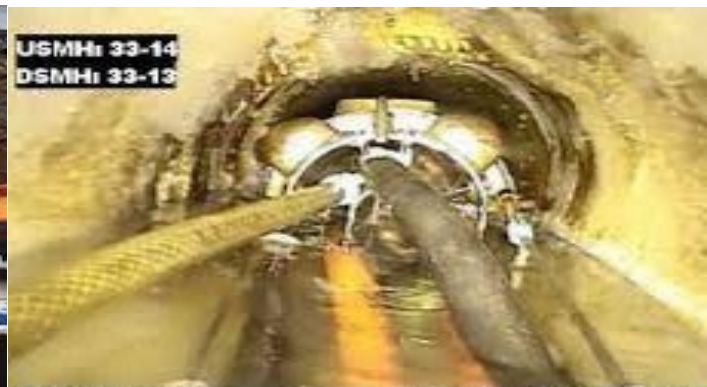
CCTV footage of Chemical Injection grouting apparatus
