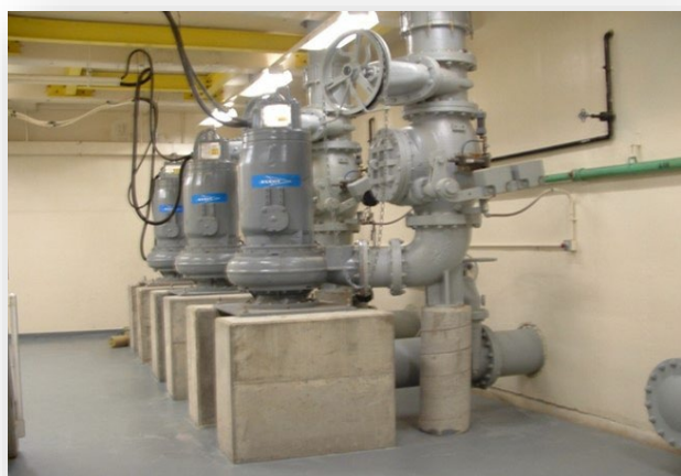
Evergreen Pump Station - Dry Pit Submersible Pumps.
