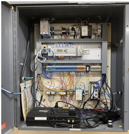
Programmable Logic Controller
