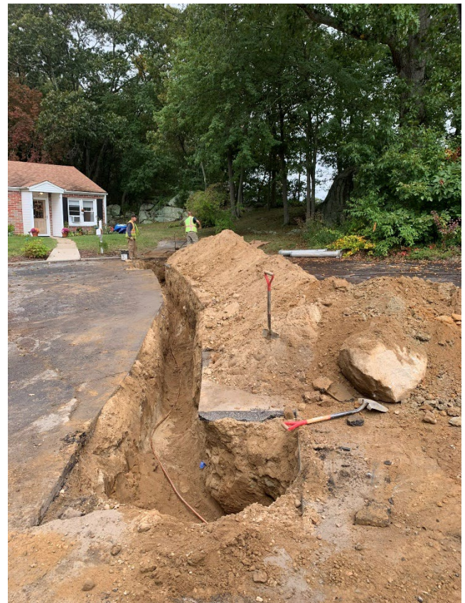
Plastic Water Service replaced with copper line
