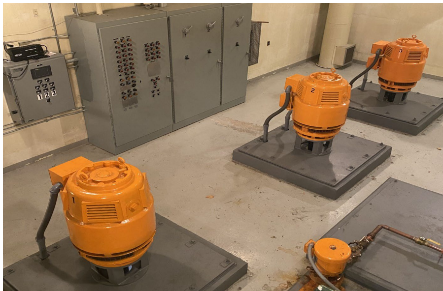
75 Horse Power Induction Type Electric Motors
