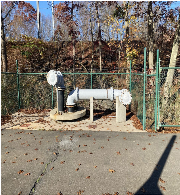
Emergency By-Pass Suction Piping
