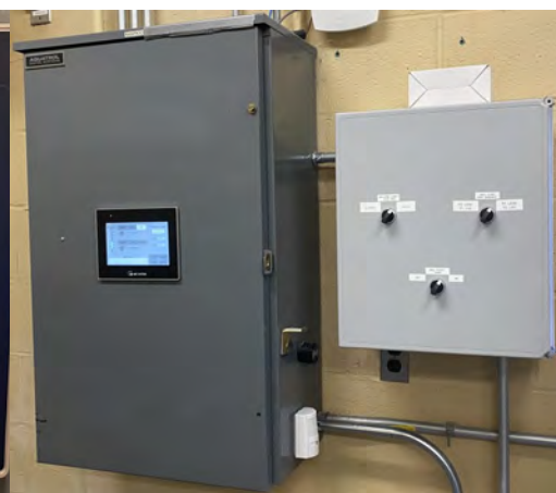
Redundant Level Control System
