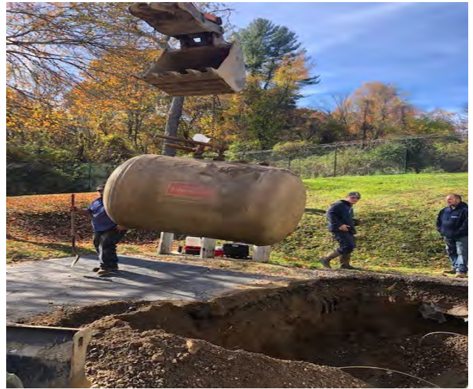
Underground Fuel Storage Tank Removal
