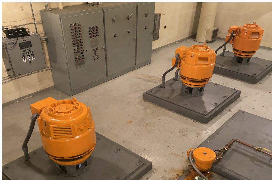
75 Horse Power Induction Type Electric Motors
