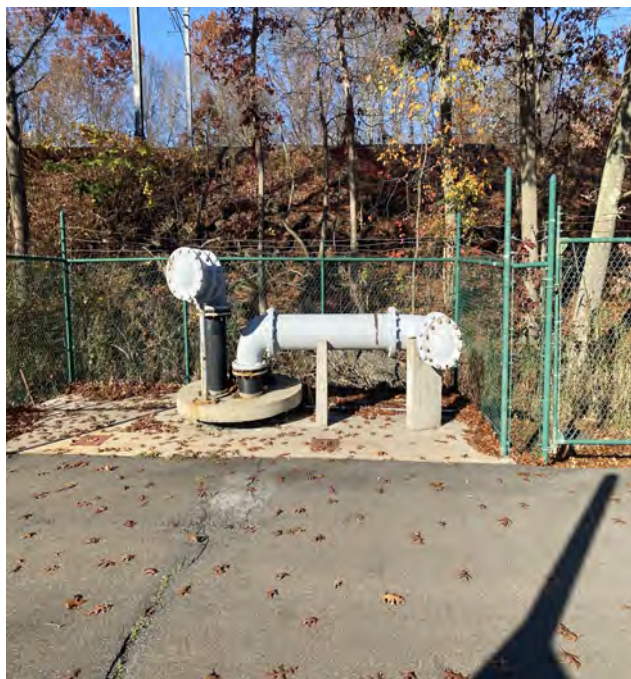
Emergency By-Pass Suction Piping
