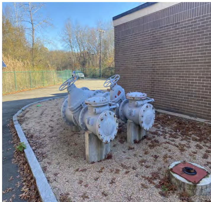
Emergency By-Pass Discharge Piping
