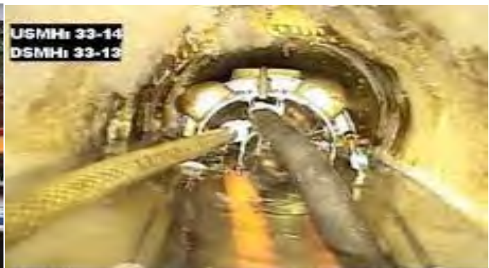
CCTV footage of Chemical Injection grouting apparatus
