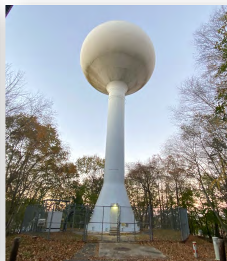
Vauxhall Street Water Tower Built 1973 - Rehab 2003 Capacity – 300,000 Gallons
