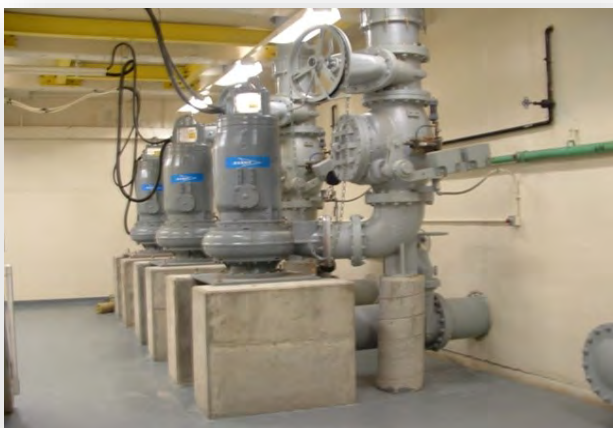
Evergreen Pump Station - Dry Pit Submersible Pumps.
