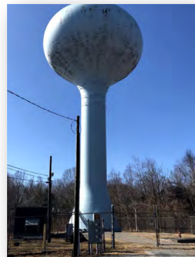
Fargo Lane Water Tower Built 1986 Capacity– 750,000 Gallons
