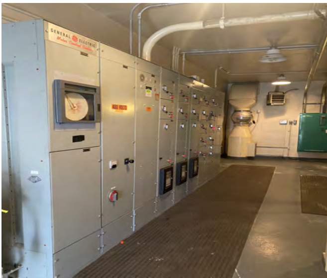
Motor Control Center and 1,000 Gallons Per Minute Centrifugal Pumps. Original equipment from date of station's construction in 1976.
