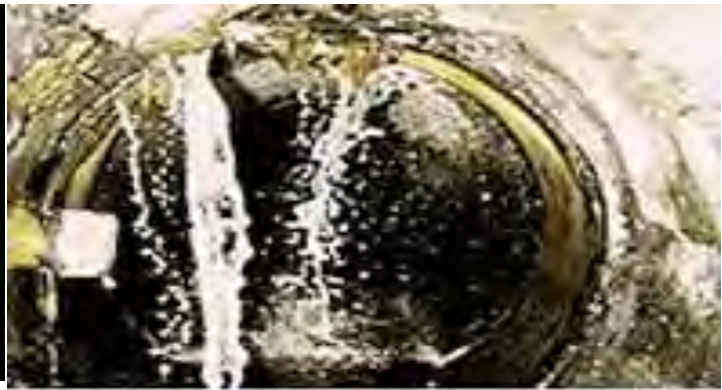
CCTV footage of Infiltration from faulty pipe joints
