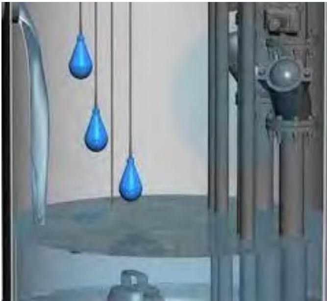
Redundant Ball Float Level System
