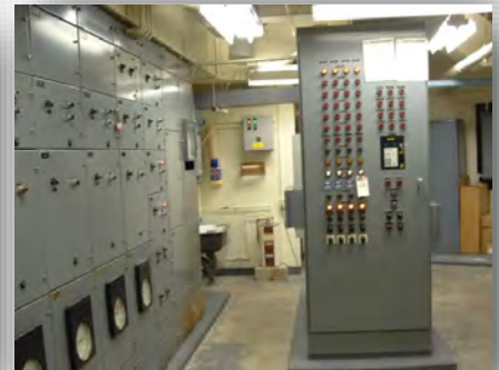
Pump station motor control panel.
