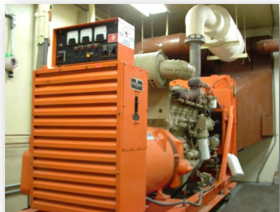
Typical Emergency Generator
