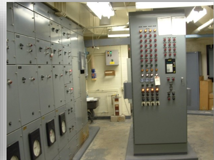
Pump station motor control panel.
