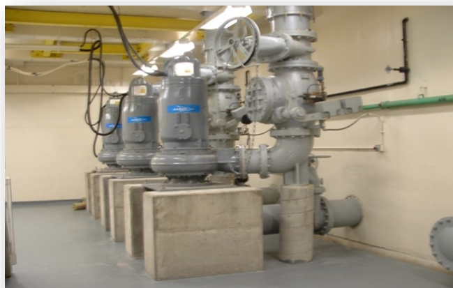
Evergreen Pump Station - Typical Dry Pit Submersible Pump.
