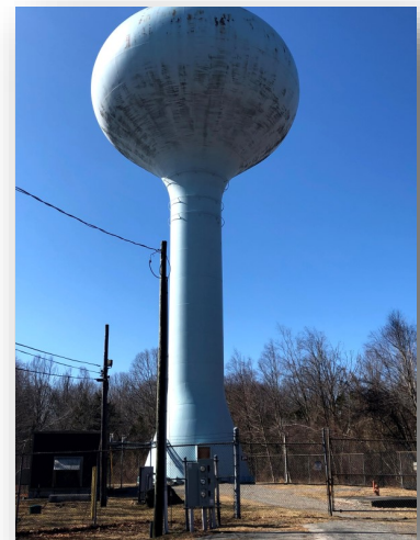
Fargo Lane Water Tower Built 1986 Capacity– 750,000 Gallons
