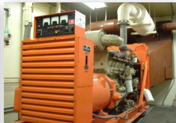
Typical Emergency Generator
