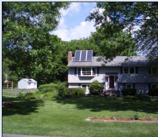
Residential Solar Collector
